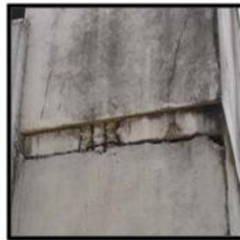
**Figure 2 :Poor Connection**
