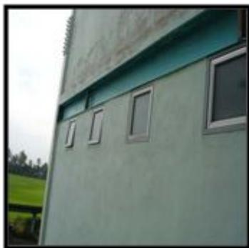
**Figure 3:Poor design steel beam exposed**
