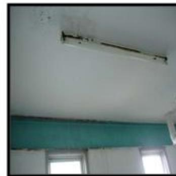
**Figure 4:Lighting system corrode**
